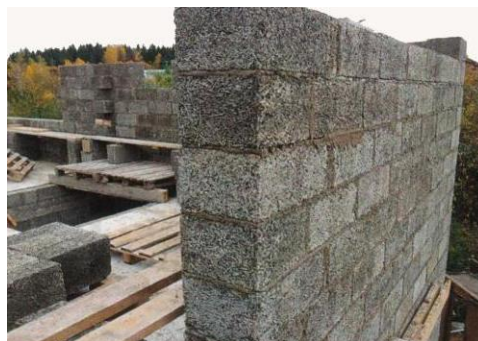
Fig. 4 – Layering of wood-chip cement-bonded blocks (Photo taken from [35][34])
