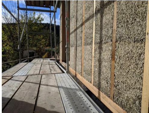
Fig. 1 – Hempcrete wall performed by tamping method (Photo taken from [32])
